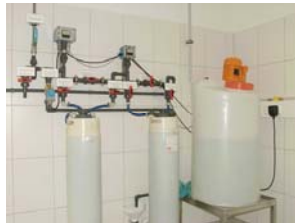
Example of a water supply with an easy cartridge change
